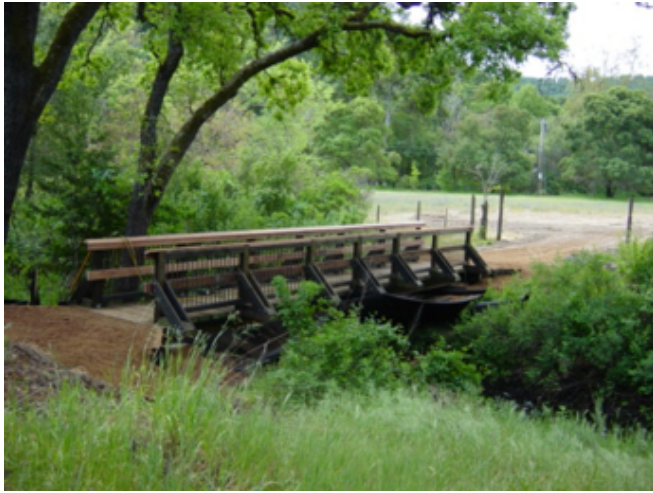
Pedestrian Bridge over Baldy Ryan Canyon Creek
