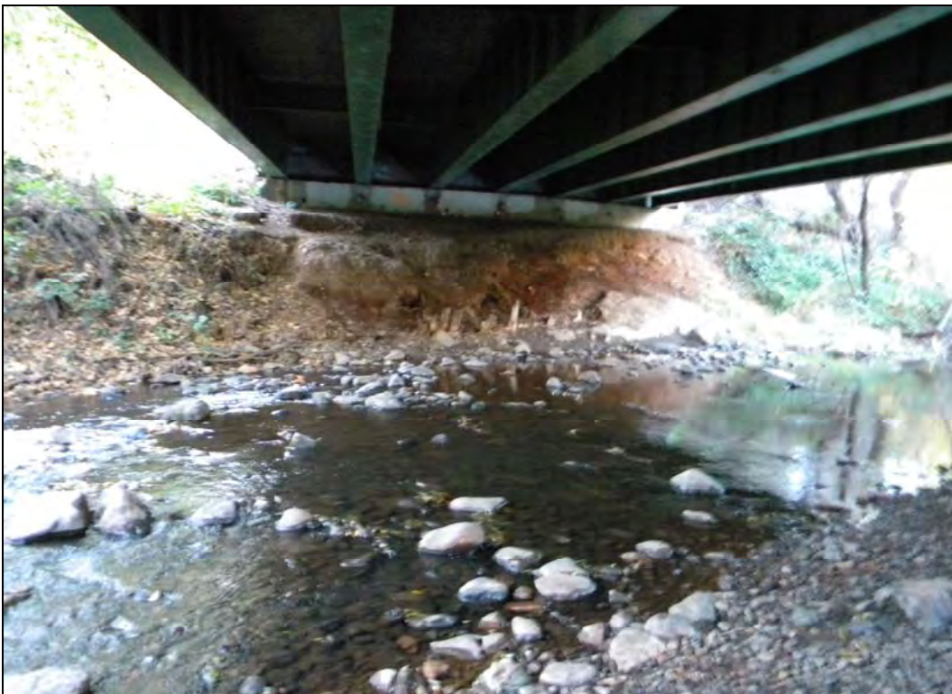
Figure 9: View south-southwest of ACB-1 with wood wall remnants
