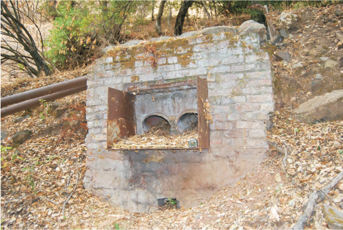
Figure 6: DG-2 Feature (view to north)
