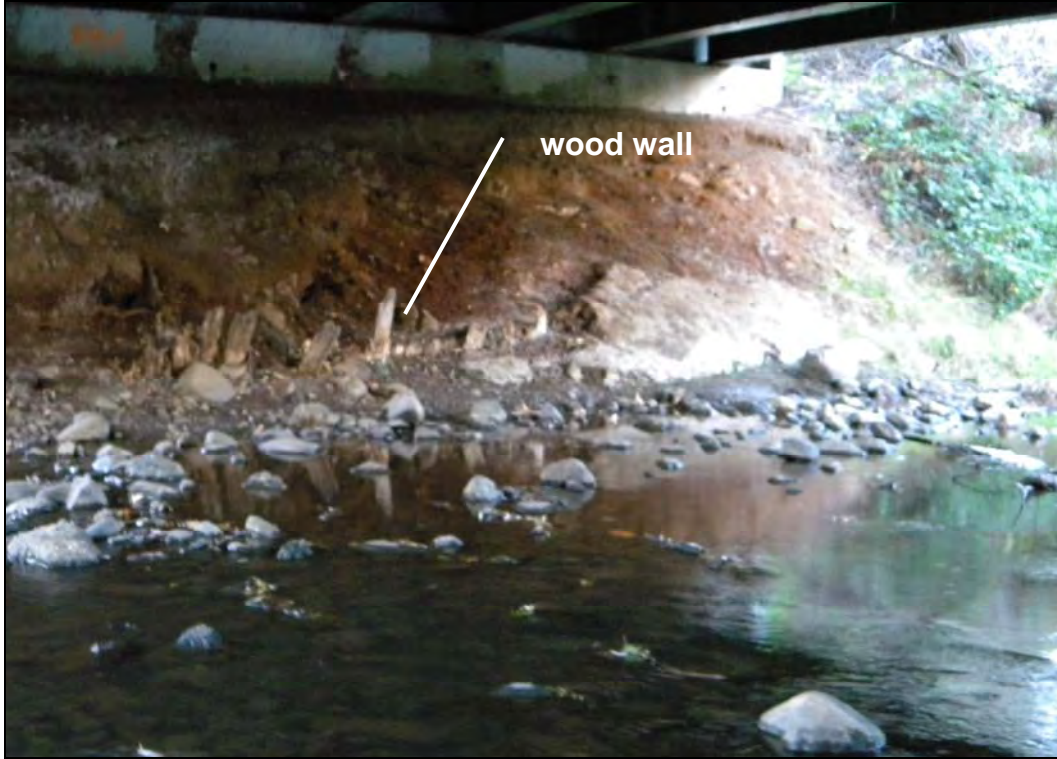
Figure 10: View south-southwest of ACB-1 with wood wall remnants
