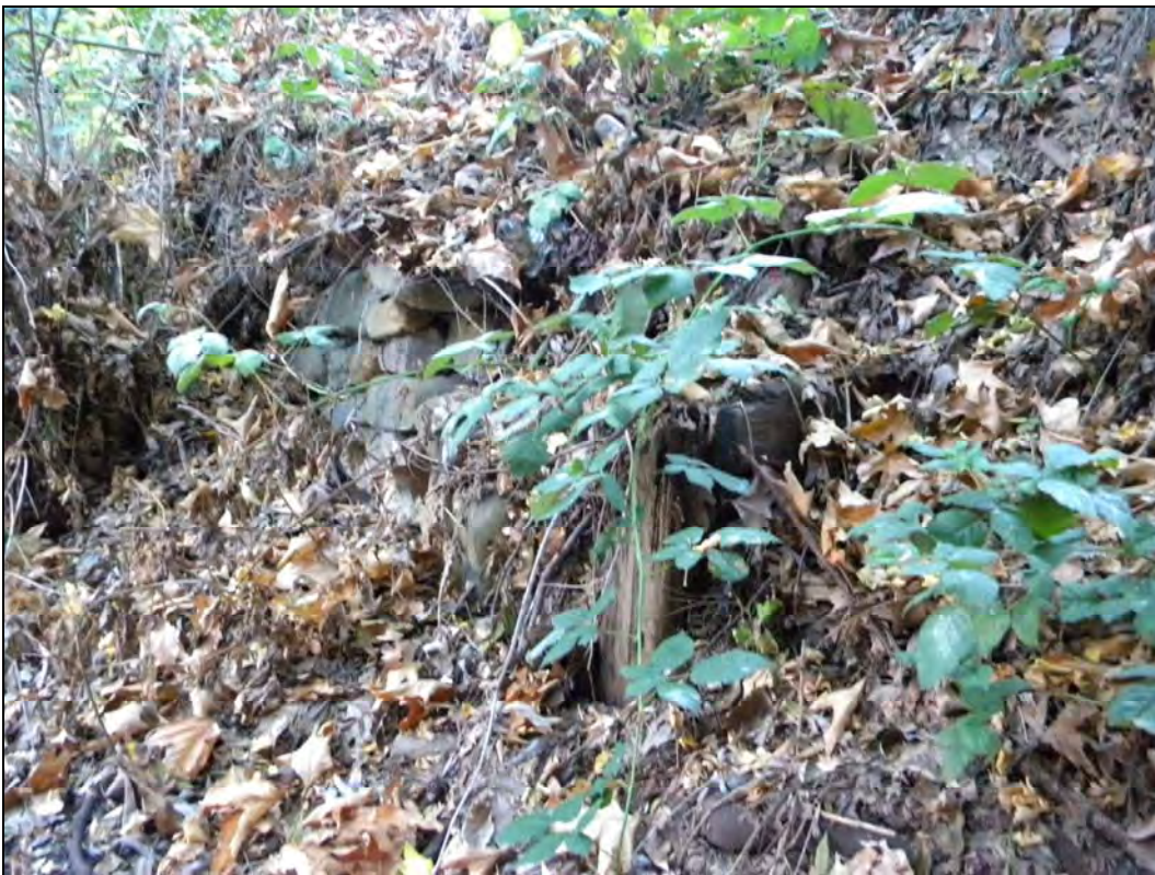
Figure 13: View east of stone wall with wood wall remnants
