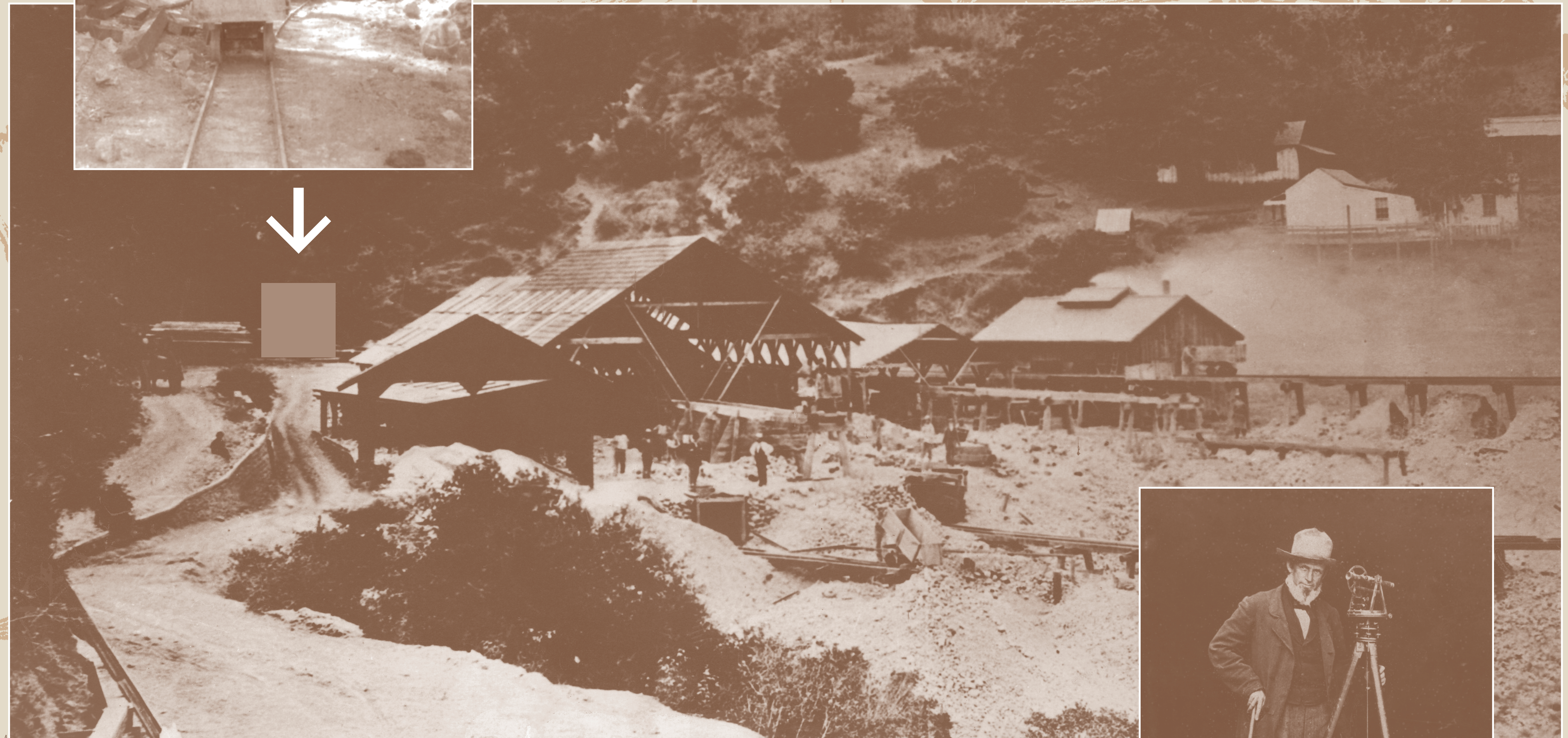
below: Day Tunnel Planilla (ore sorting shed), ca late 1800s
