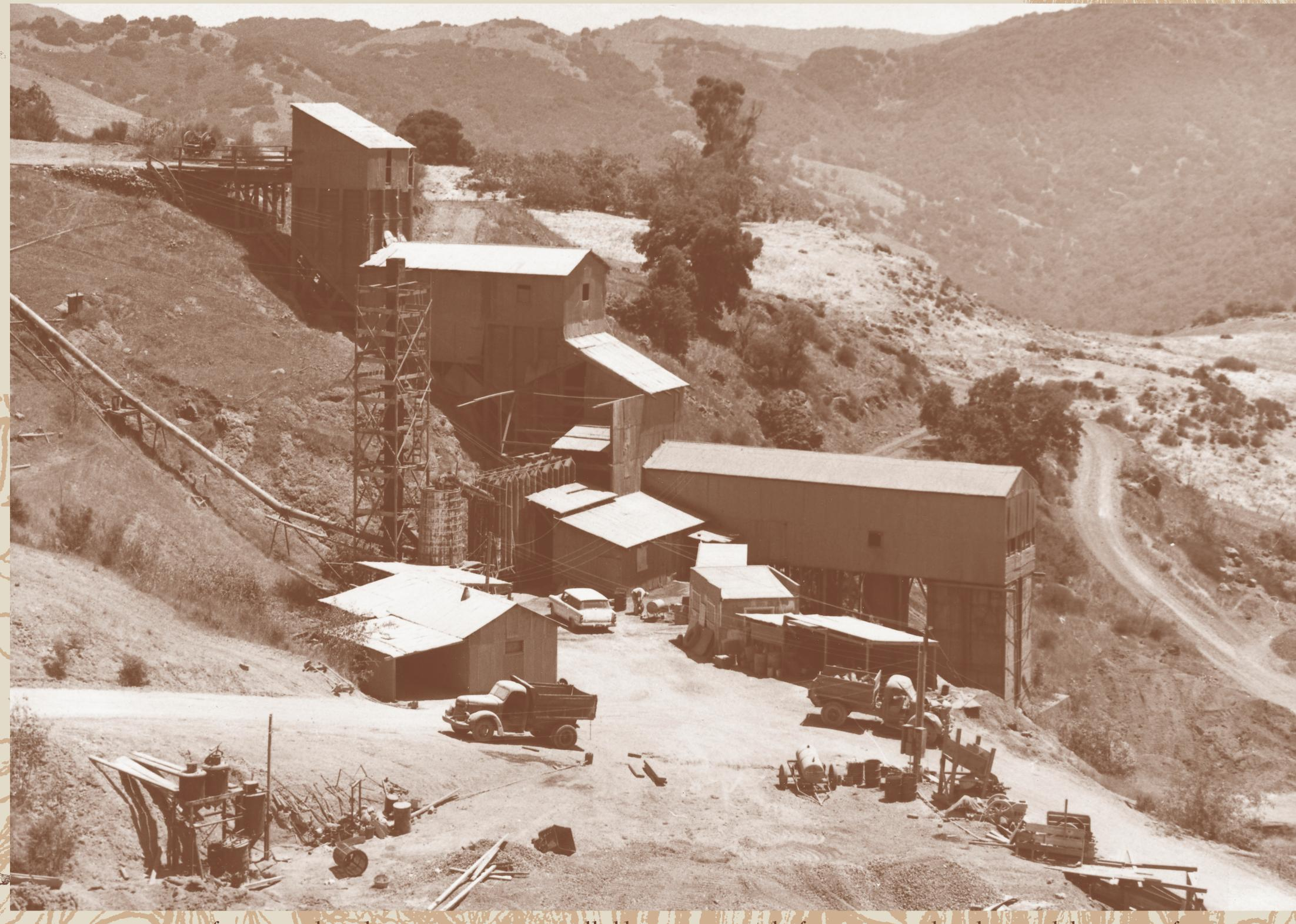
A 100-ton rotary furnace and condensing system was installed here in 1940. The furnace proved too large and this 50-ton furnace, which worked best when processing about 35 tons of ore, replaced the first one. Gould's furnace technology brought the New Almaden Mines into the 20th century, winning worldwide recognition for productivity. This furnace was used until 1976, when the property was purchased by the Santa Clara County Parks Department.
