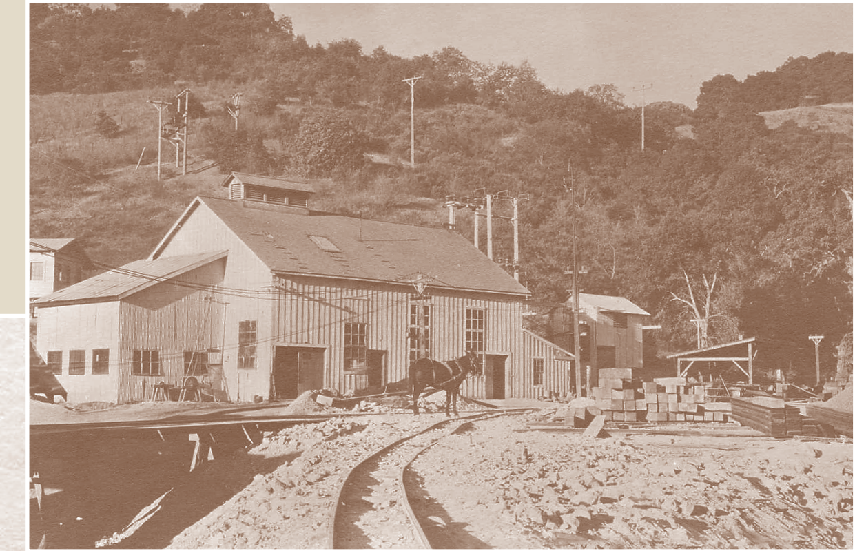
Senador Shop circa 1916. The mule was used to haul ore, timber and equipment in and out of the mine. The mine's heyday was 1915 to 1926 although it was worked on and off from 1863. The barn was dismantled in 1940 and moved to the English Camp site at the New Almaden Mine and is still there today.
