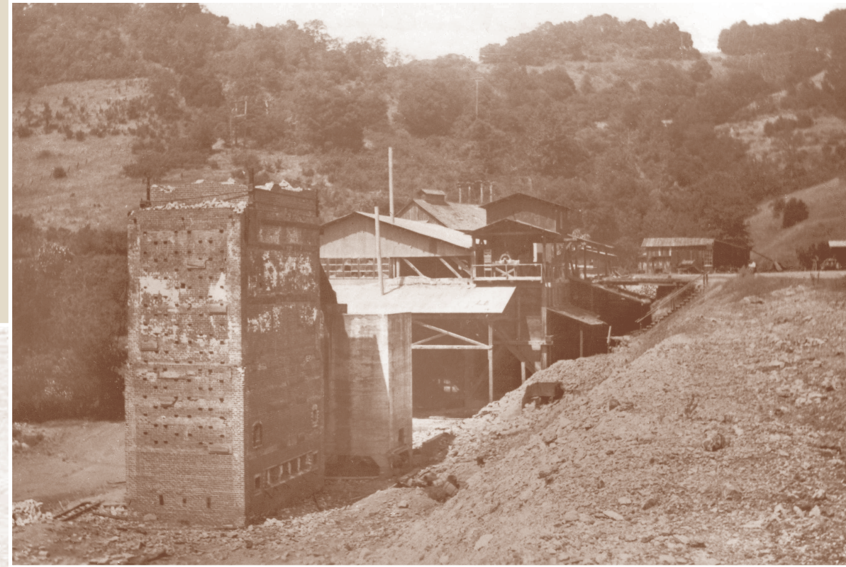
The two concrete towers are dust bins from the old 90-ton-per-day Scott Furnace Plant.
