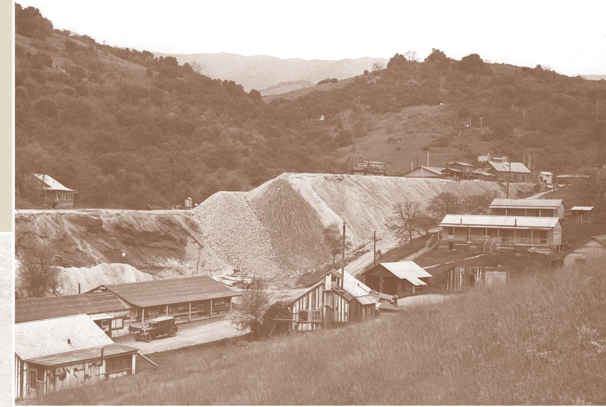
El Senador Mine circa 1924, looking west towards the Senador Trail. The Furnace plant is barely visible behind the dump of waste rock (right), burnt ore (middle) and furnace dust (left).
