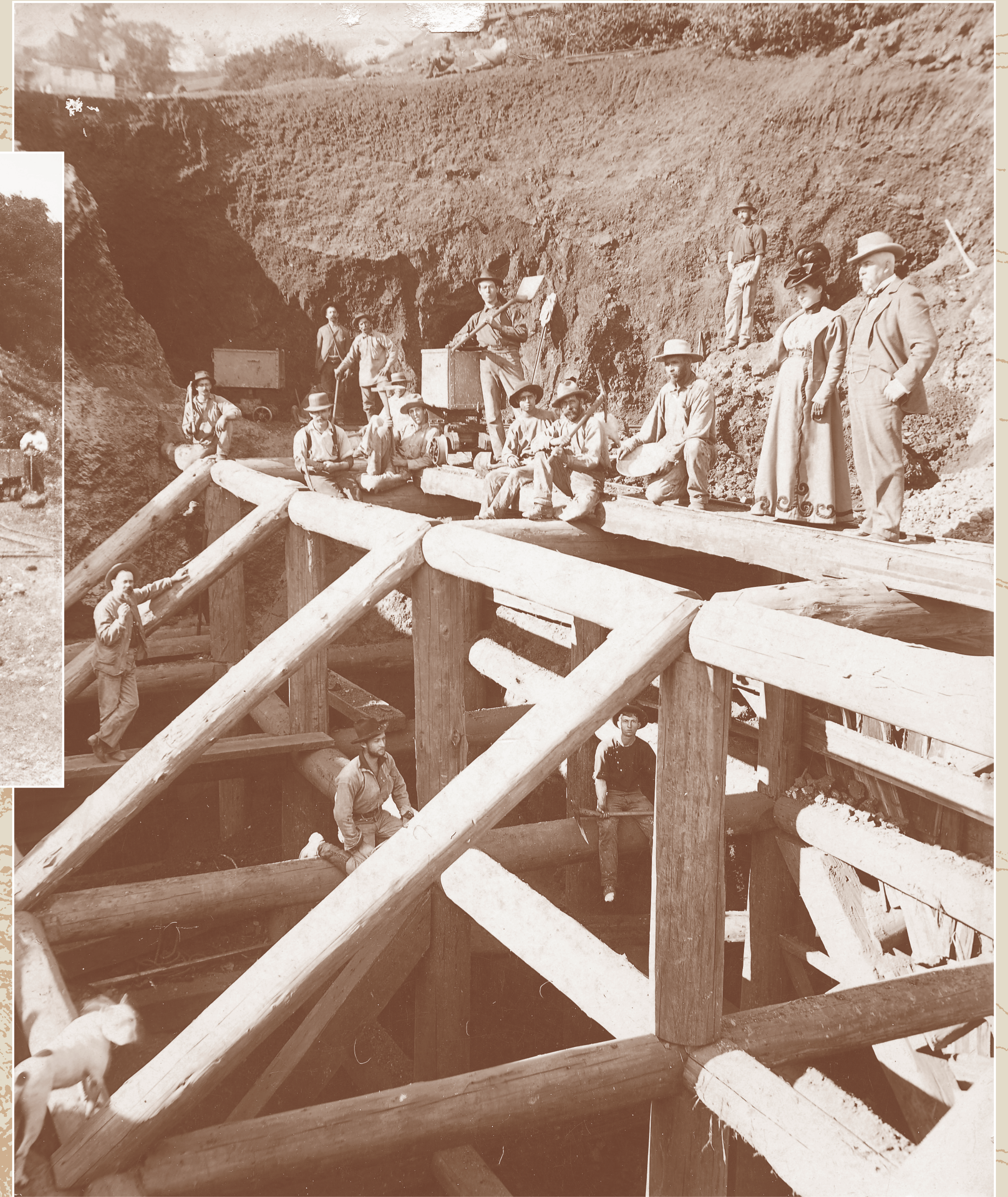
Mr. Derby, the mine company storekeeper, and Mrs. Derby inspect the opening of the Yellow Kid's west portal.
