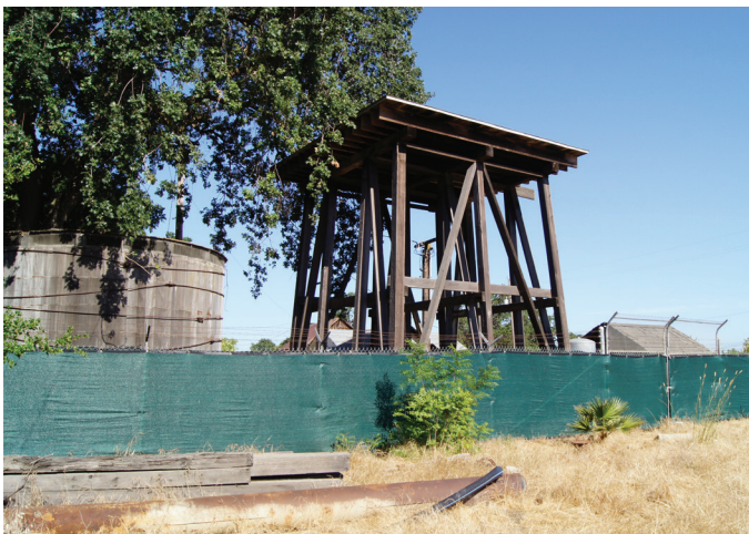
Photo of the Water Tower
