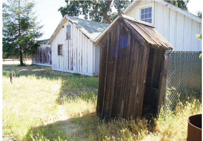
Photo of Outhouse Building
