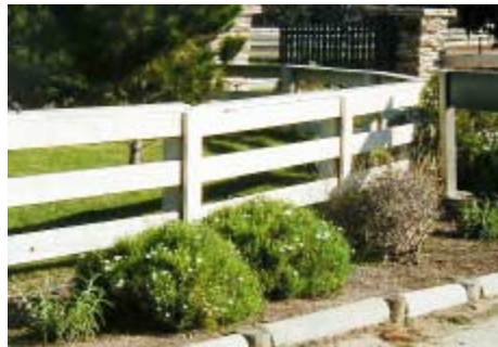
Corral Fencing with Wood Curb and Planting
