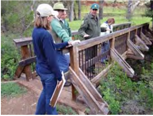
① Low impact span bridge across creek on existing multiuse trail
