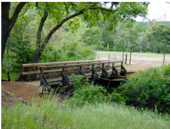
Pedestrian Bridge over Baldy Ryan Canyon Creek
