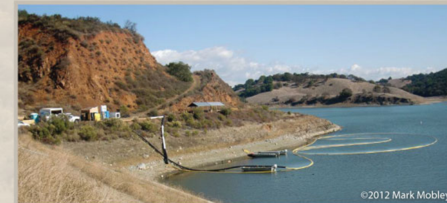
Aeration system in Calero Reservoir.
