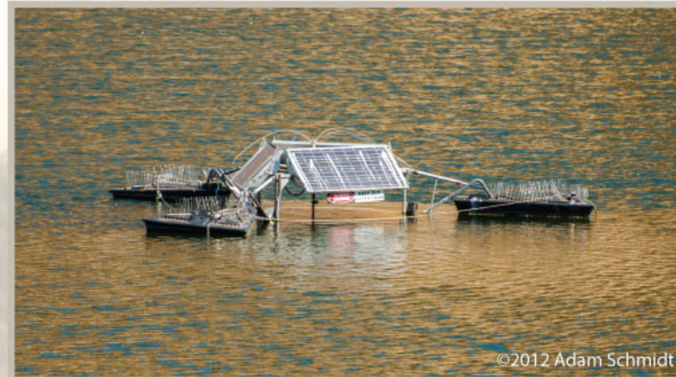
Water circulator in Almaden Reservoir.
