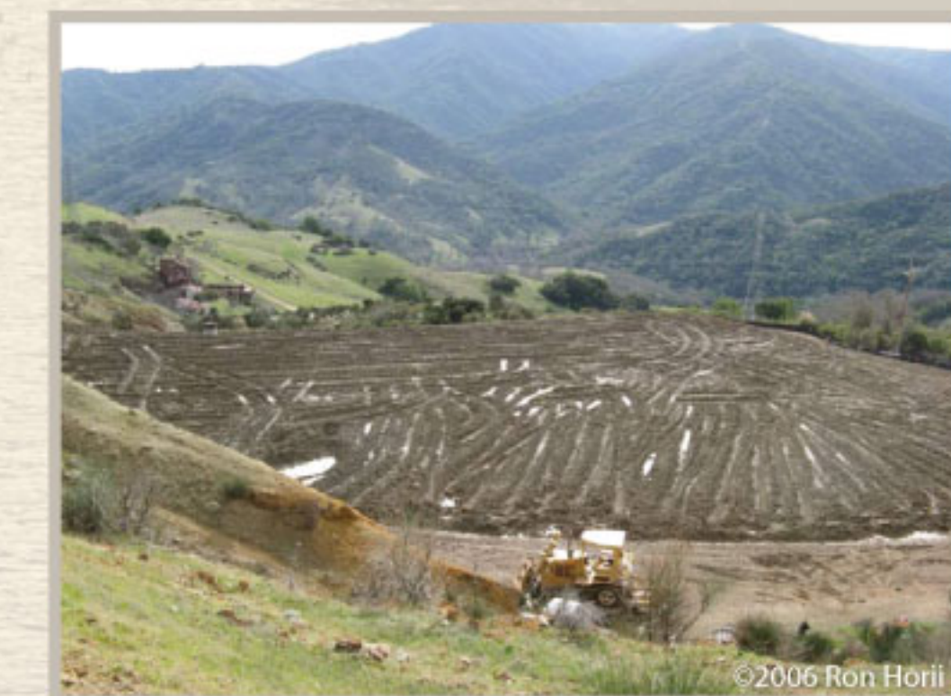
Mine Hill, San Francisco Open Cut.
