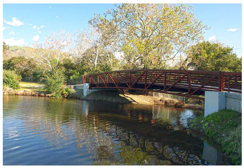
Bridge along Penitencia Creek
