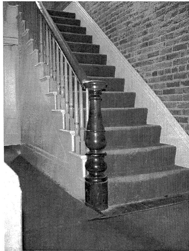
Main Stair Railing
