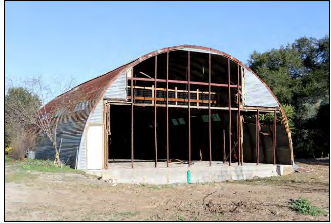
Photo 13. Metal Quonset structure at the Ranch Complex Area.
