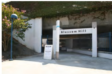
Entrance to Blossom Hill light rail Station
