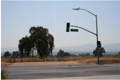
Existing signal on Branham Lane
