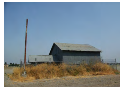
Existing pump house
